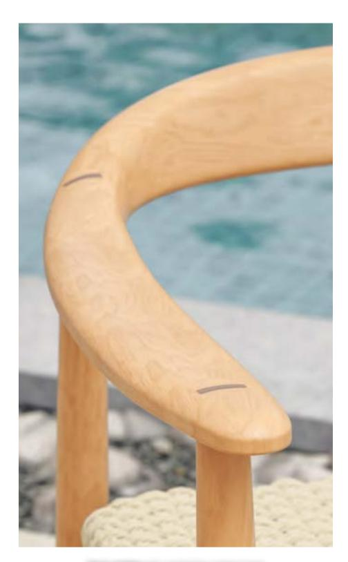
Tenon wedges with contrasting colored wood securely attach the armrests to the lathe-turned legs.
