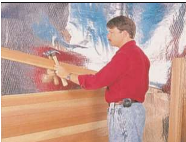
Installed on framing; vapor barrier between studs and T&G on warm side of wall.
